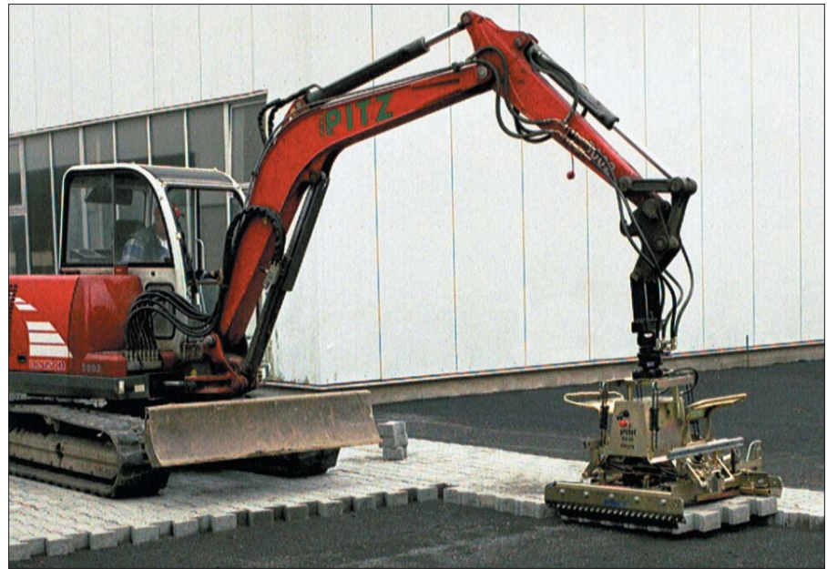
Pushing Off Device (ADV) – No Realignment – Joints Always Comply with the Regulations
